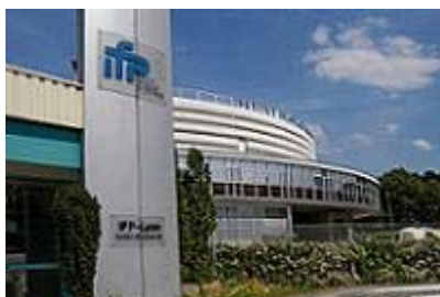
Facility in Lyon, France, IFP
